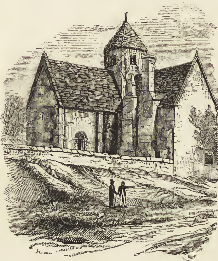
63. Penmon Church, Anglesey. Norman central Tower.
